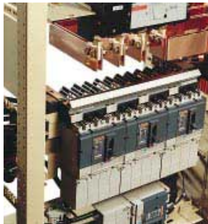
Fixed, vertical Compact NS100/250 circuit breakers connected to the busbars by the Polypact distribution block. The distribution block is supplied with prefabricated connections and a barrier that secures the conductors and implements Form 2 separation.
