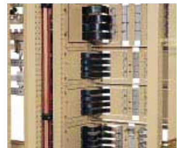
The connection is supplied with a barrier that secures the conductors and provides Form 2 separation.
